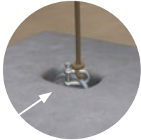
Anchor rope to anchor block connection
